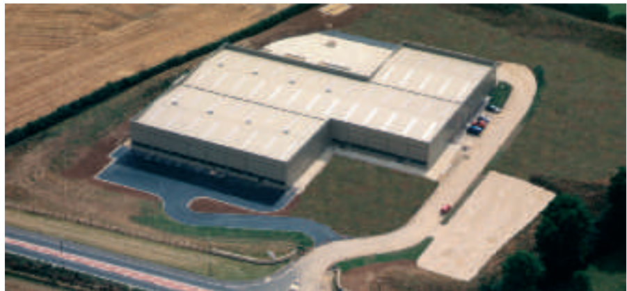
Autogard's modern plant at Cirencester, England
